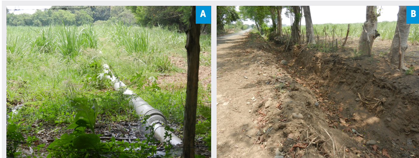
Figure 19 A) Transport of pumped water from Río Paz to the cane field (April 2019, N13 47.480, W090 06.941). B) Diversion of the Aguacate River by digging ditch with an excavator to irrigate the cane fields (April 2019, N13 46.540, W090 05.572).
